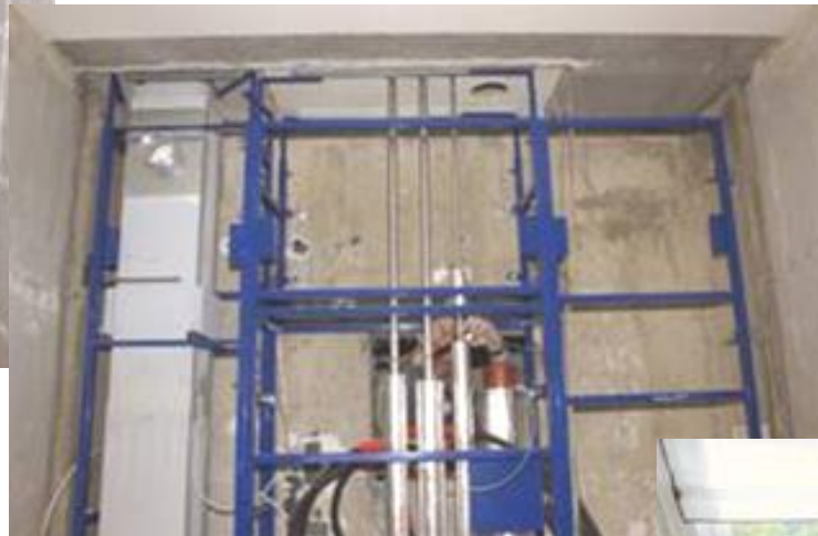
... on the exchange of the old pipelines ...
