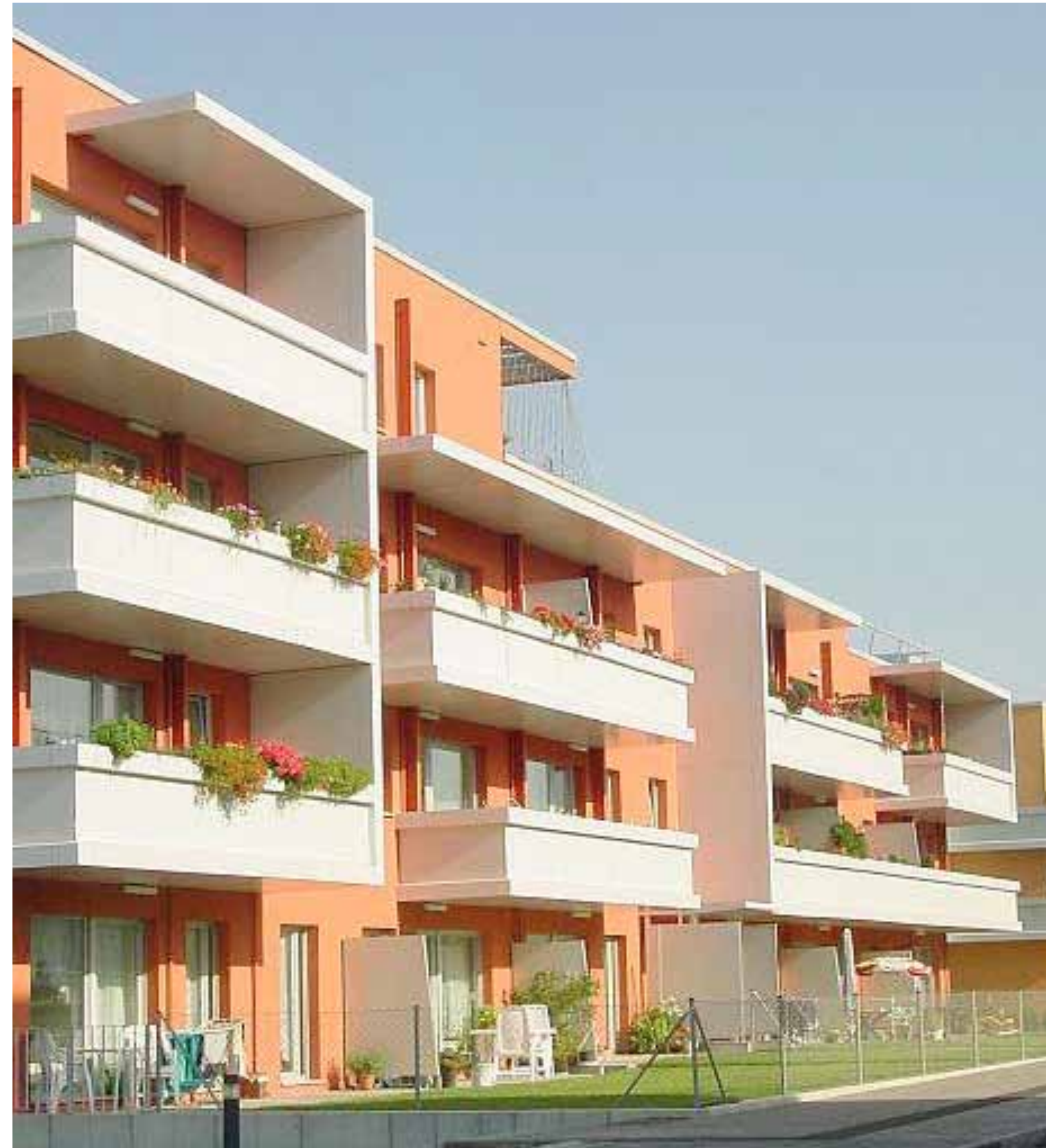
05. Fully refurbished building in Dresden Gorbitz
