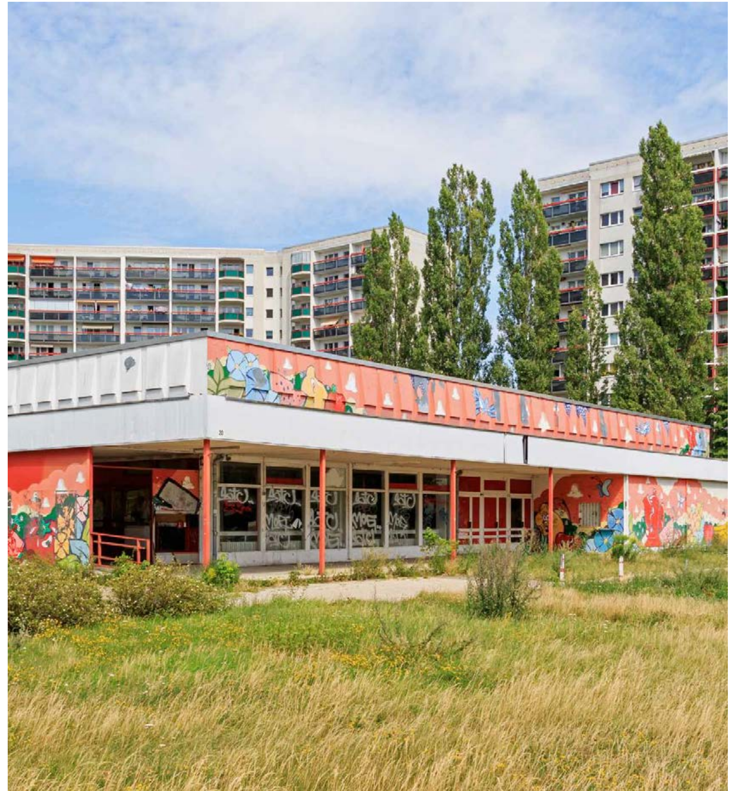
09. Large settlement Berlin Marzahn Ahrensfelderterrassen
