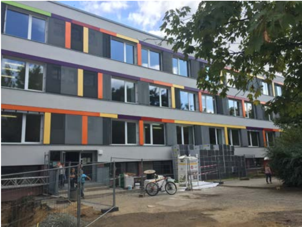
school renovation in Gorbitz, Dresden
