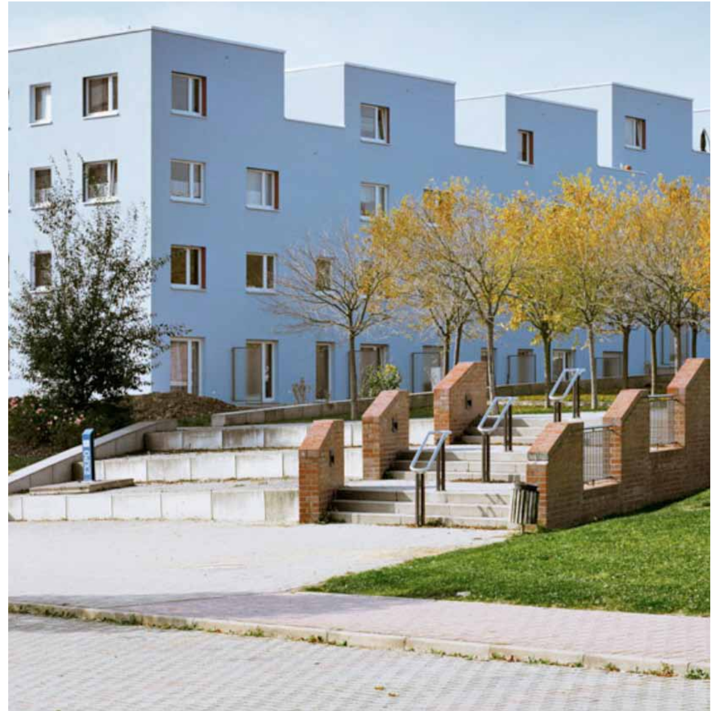
11. Leinefelde before and after transformation
