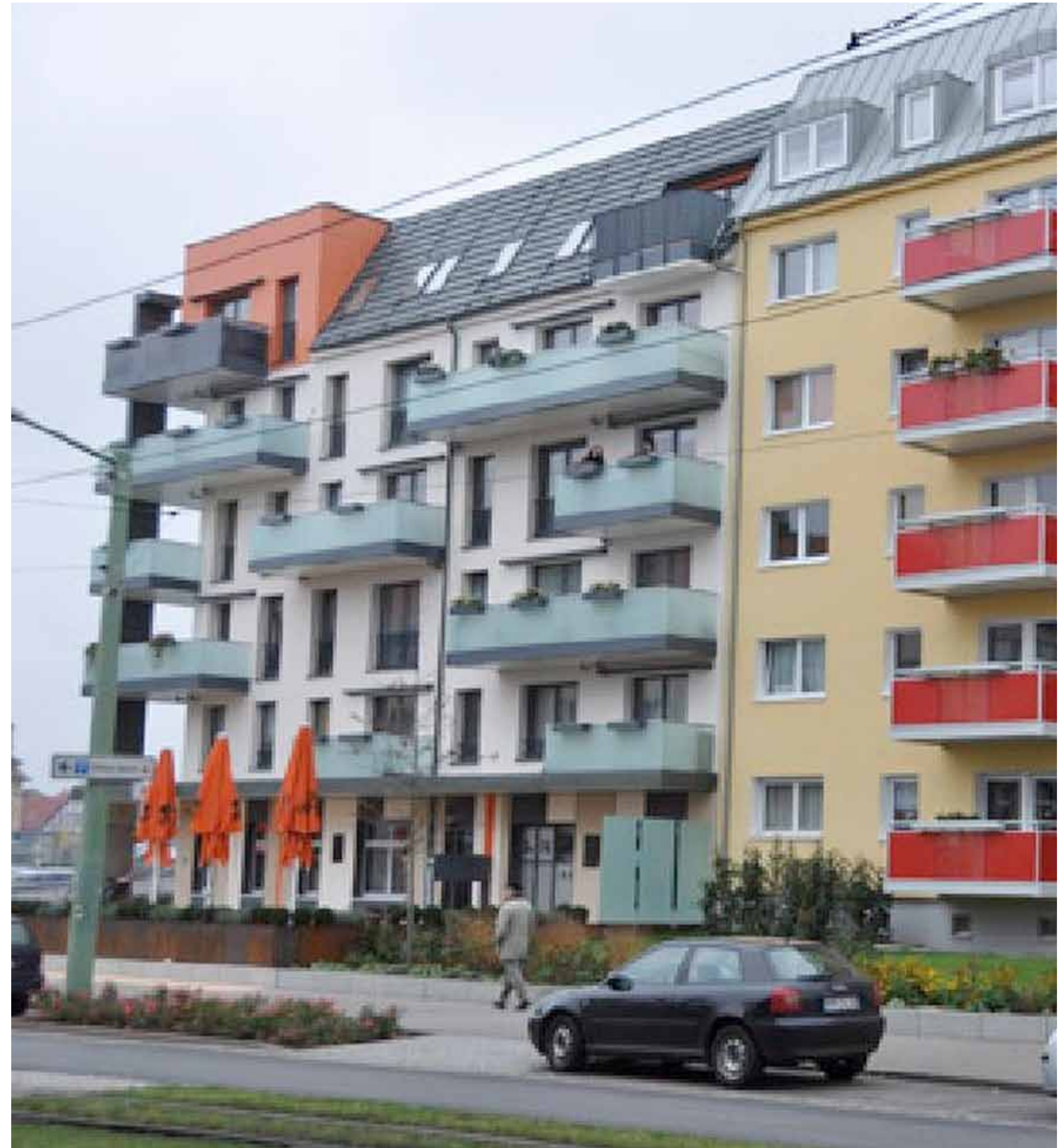
08. Buildings with new balconies, new insulation
