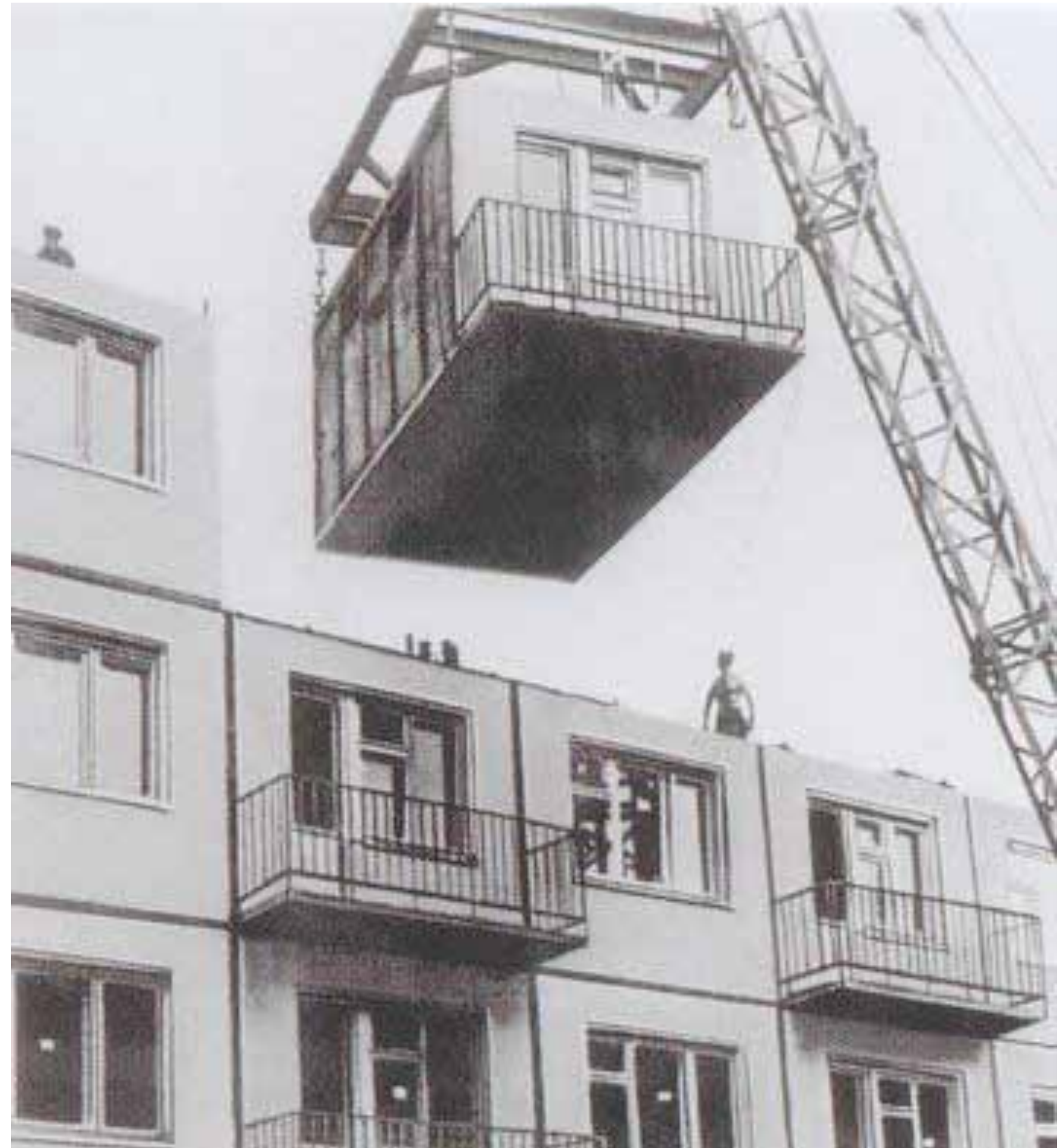
17. Instalation of prefabricated Unit
