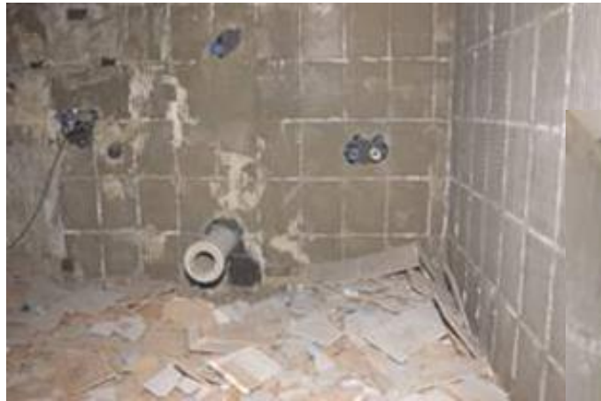
From the demolition of the old bath ....
