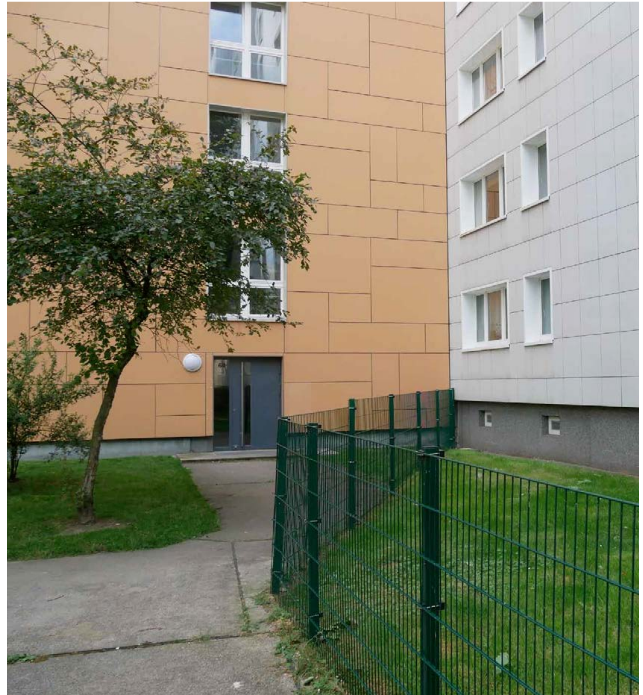
27. Fence as evidence for new ownership
