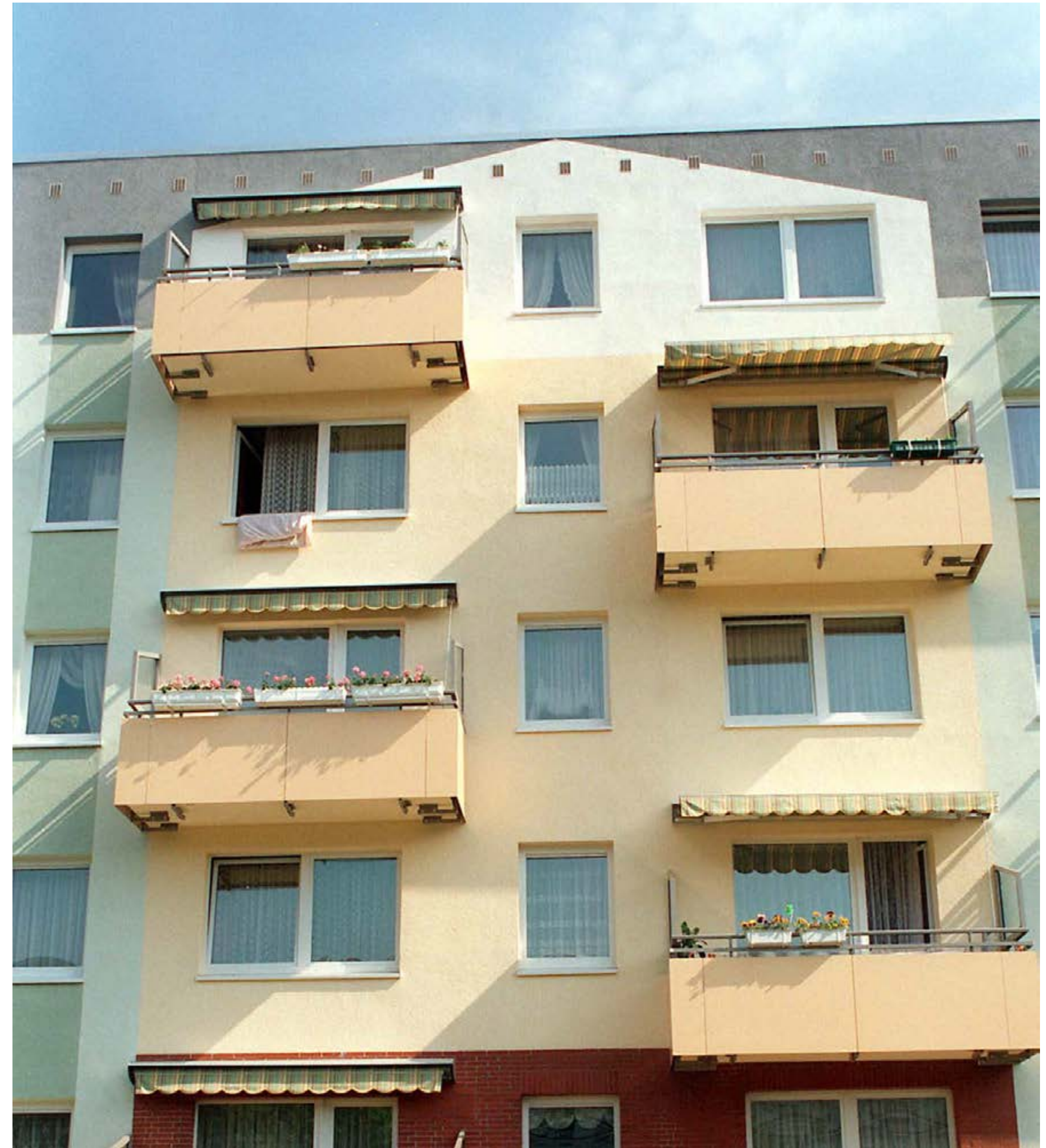
07. Aesthetically renovation painted of slanted roof
